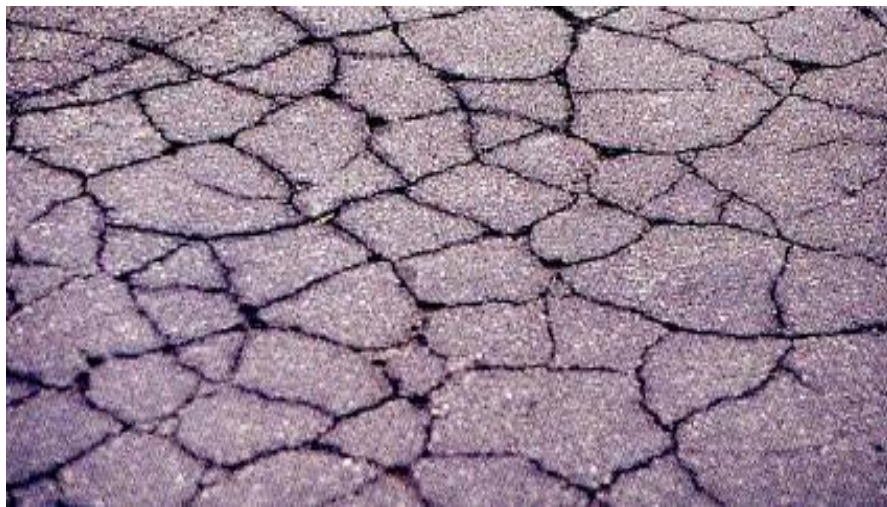
Figure 1. Fatigue cracks in asphalt pavement
